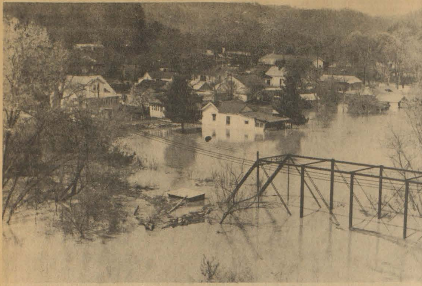
PHOTO SHOWS widespread flooding in the West Prestonsburg vicinity.
