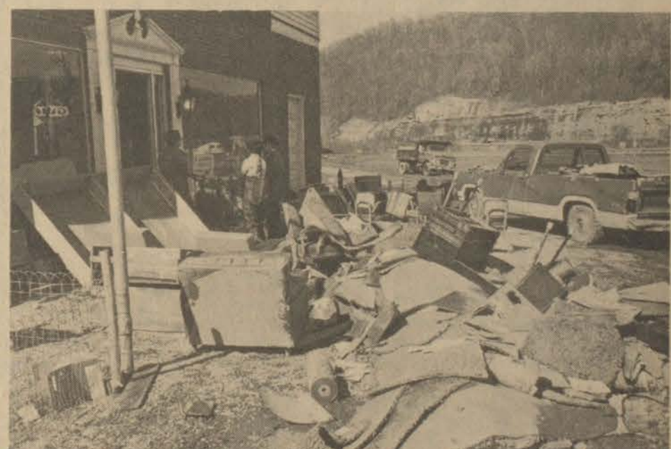
THIS SCENE FRIDAY at the accounting firm of W. Luginbyhl & Associates here was repeated hundreds of times throughout the county as merchants and businessmen dug out of the muck.
