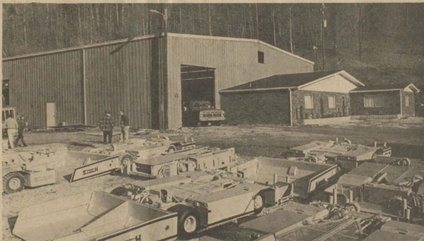
Buildings and grounds of S. & H. Manufacturing Company on Brush Creek. Motorized mine scoops are pictured parked in foreground.
