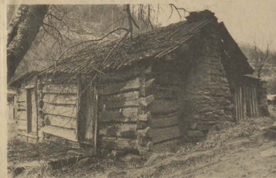
LOG HOUSES such as this abandoned structure on the Beech Branch of the Left Fork of Middle Creek are vanishing reminders of this mountain section's not so far removed pioneer past. This cabin is particularly true to the "old" style with rived-board roof, mud "chinking", and double doors constructed of broad planks.
