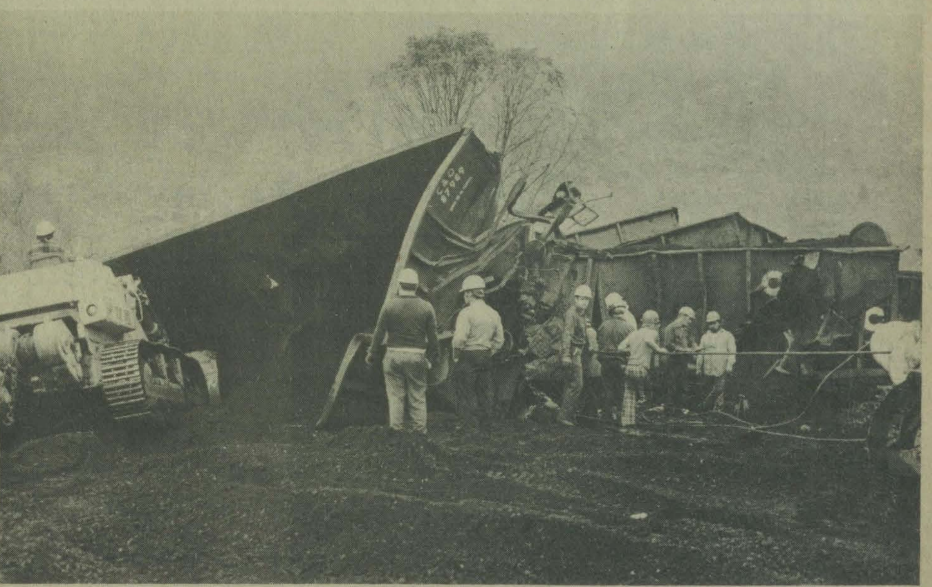
Dozers and other heavy equipment at work at Allen, scene of 18-car derailment, moving coal spilled from gondolas and clearing wrecked cars from the right-of-way.
