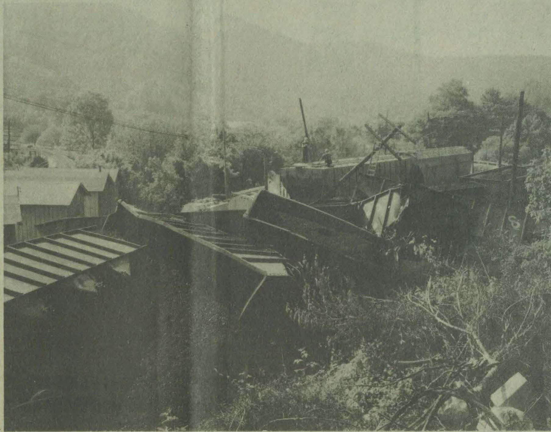
This train wreck, one of several experienced by the C. & O. in recent months, took place at 7:15 a.m. Tuesday, opposite the town of Allen. Nine loaded coal cars, moving out of Beaver Creek to market, were wrecked and a long stretch of rail was twisted. Nobody was hurt. There was no estimate of the damage, and rail officials said the investigation of the wreck had not progressed to the stage that they could fix the cause.
