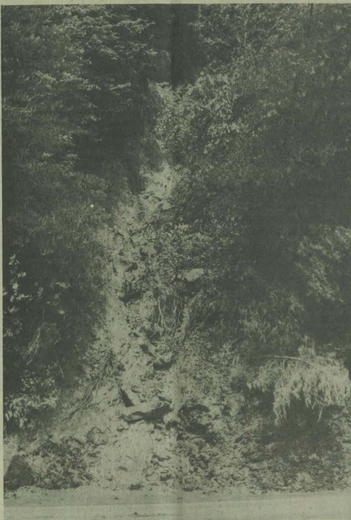
Rain, which over the week-end resulted in extensive loss of property and two lives in neighboring Pike and Letcher counties, caused minor damage in Floyd. In the Prestonsburg vicinity, this mudslide, which covered U.S. 23 near the Ball Alley curve for a time Saturday, held up traffic for hours.
