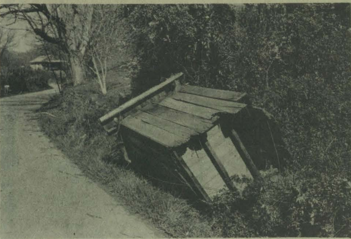
Monday night's "twister" was also rough on outdoor plumbing, as evidenced by this Abbott Creek facility which was upended by the storm and dropped to the side of the road. Luckily, the structure was not occupied at the time.
