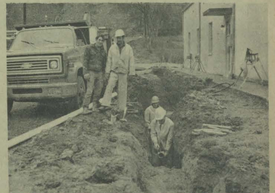
Telephone company employees at work on underground cable here.
