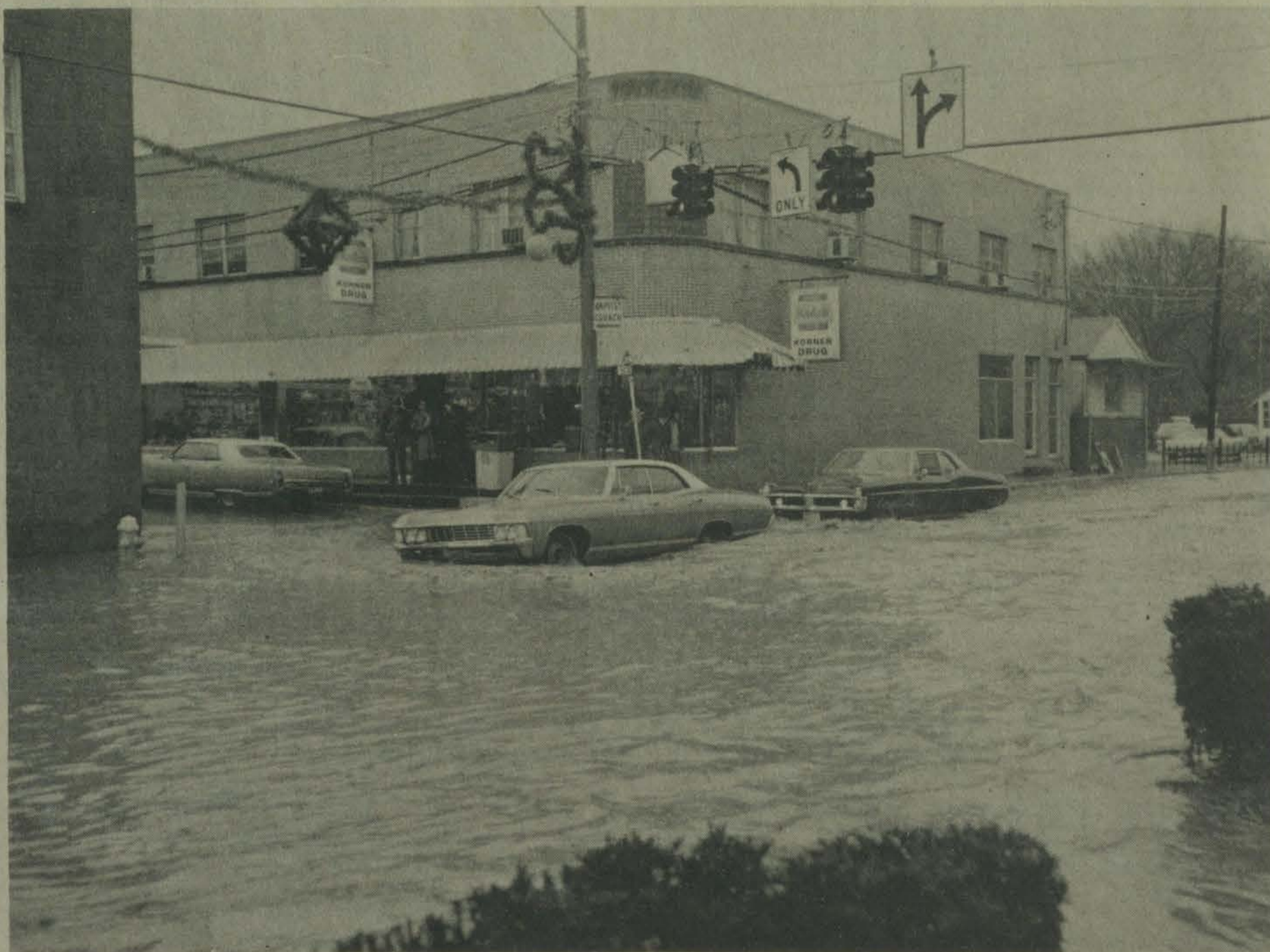
This scene, reminiscent of earlier days when the Big Sandy flooded Prestonsburg, was created Tuesday morning when the runoff of water during a heavy rain overtaxed drainage facilities at the Lake Drive-Court Street intersection.
