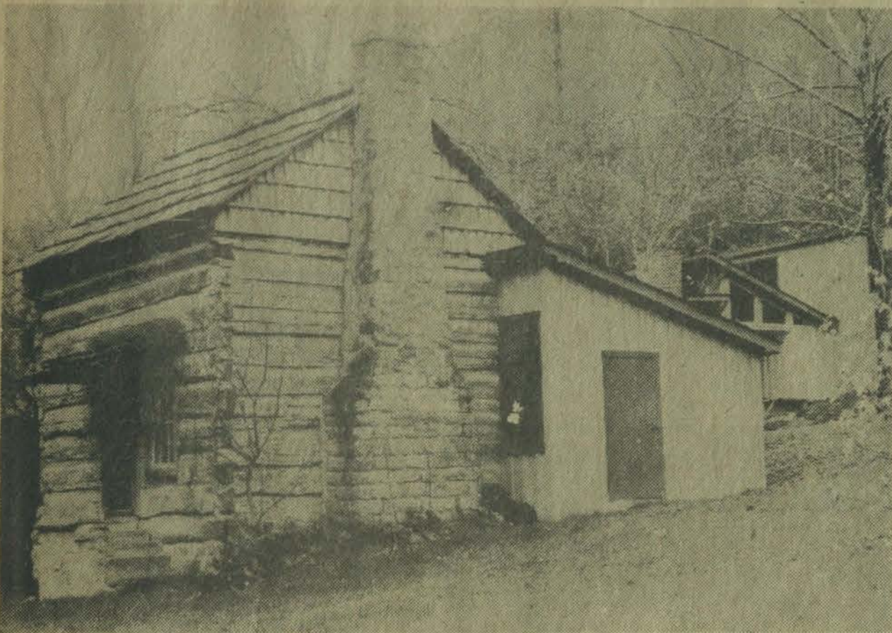
SOL EVERIDGE CABIN—Still standing at the Hindman Settlement School in Knott County is the log cabin home of Solomon Everidge, the 80-year-old pioneer who walked barefoot 22 miles to secure "learnin'" for the youth of his mountain community. The new addition to the cabin is the office of the unique school on Troublesome Creek. (Karen Tam Photo)
