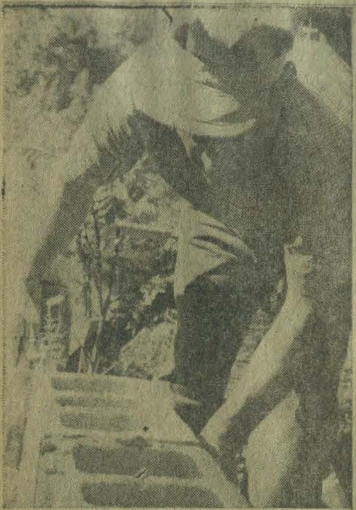
Building a pump house adds a sense of usefulness to a days work for project repair crews. Crew members must be area residents 52 or older and previously unemployed.
