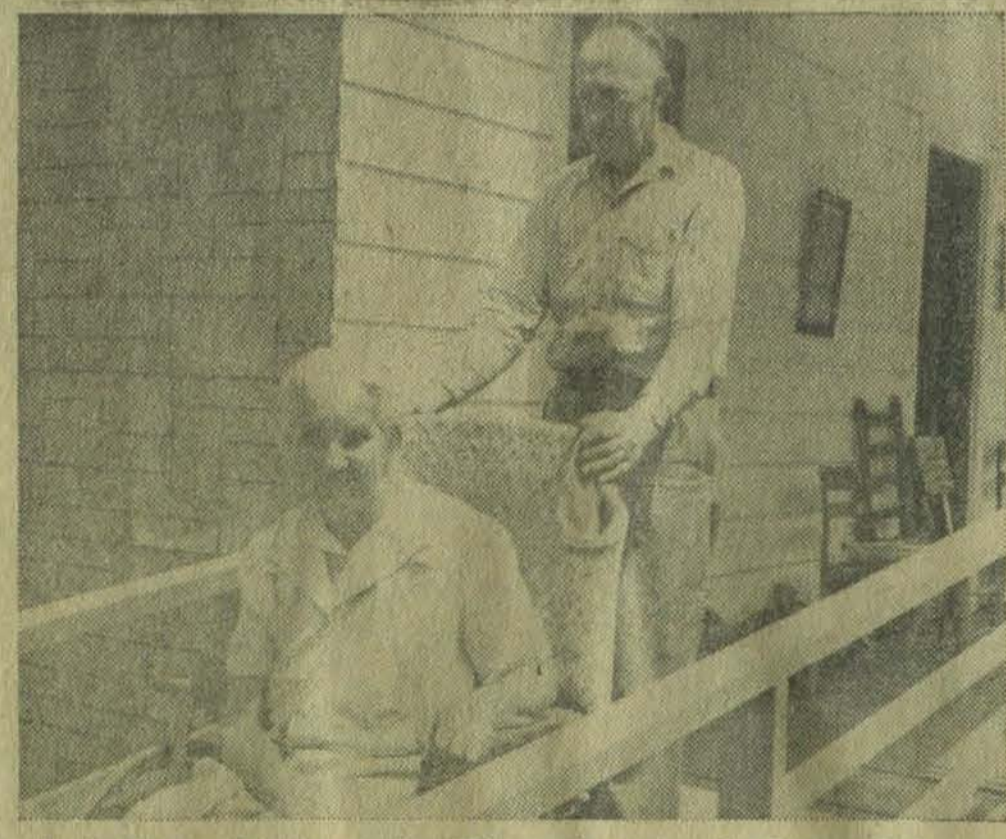
A simple wood ramp makes life much easier for Roy and Anna Ward. The construction crew built the ramp and railing while repairing the Wards' house.
