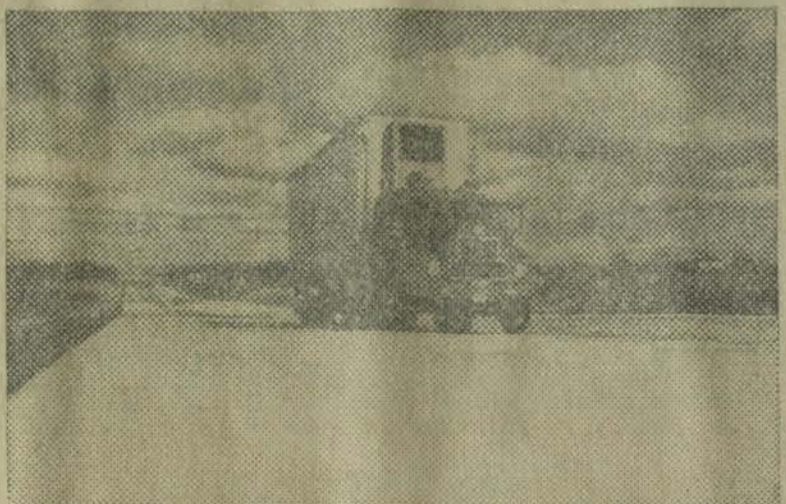
Modern Concrete Highway in Kentucky.
