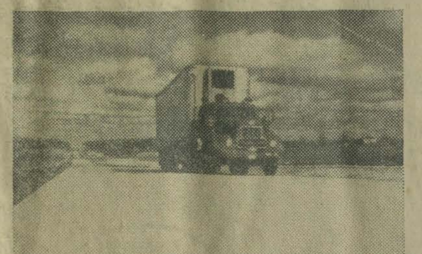
Modern Concrete Highway in Kentucky.
