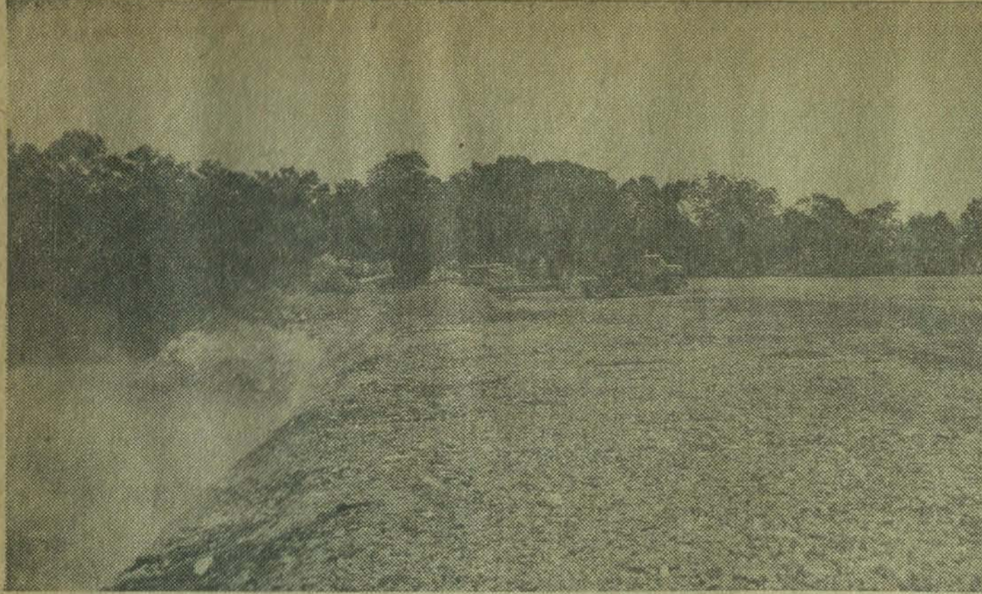
PROPER SANITATION —The Kentucky Department of Health is launching a three-year program to rid the state of unsightly and unsanitary municipal garbage dump sites and replacing them with properly operated land-fill dumps such as this one at Fort Knox — the only one of its kind in Kentucky. The area right in the picture has been filled and left in a sanitary condition.
