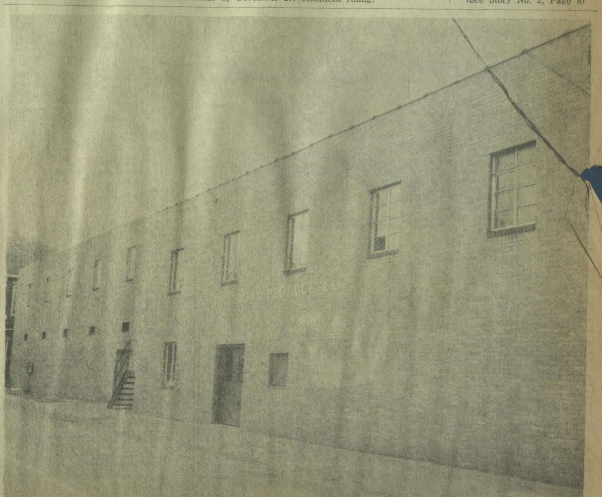
PRESTONSBURG'S LARGEST PRIVATELY OWNED BUILDING—The Brown Produce Company's Third street structure with its huge, new addition.
