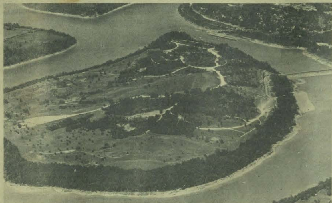
Surrounded by beautiful Lake Cumberland, Burnside Island State Park is reached by a paved causeway. A beach, nine-hole golf course, picnic area and shelters, and tent and trailer parking are in the park, which is located at Burnside near Somerset.
