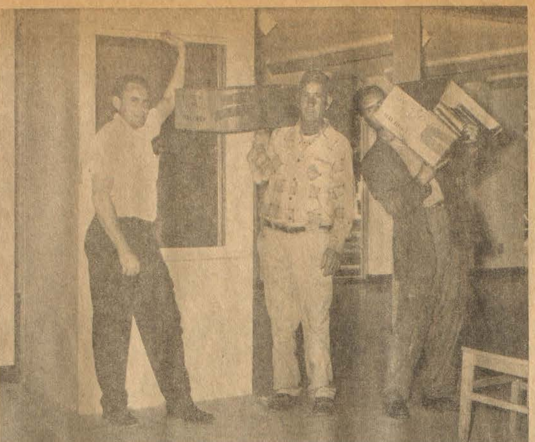
MOVING DAYS FOR LIBRARY. Charles Patton, county librarian, stands at left as workmen move some of the 30,000 books in the old Floyd County Board of Education to the new Floyd County Library nearby. The new structure, probably the finest of its kind in Eastern Kentucky, is now open to the public. Its formal dedication will be held Sunday, November 22.
