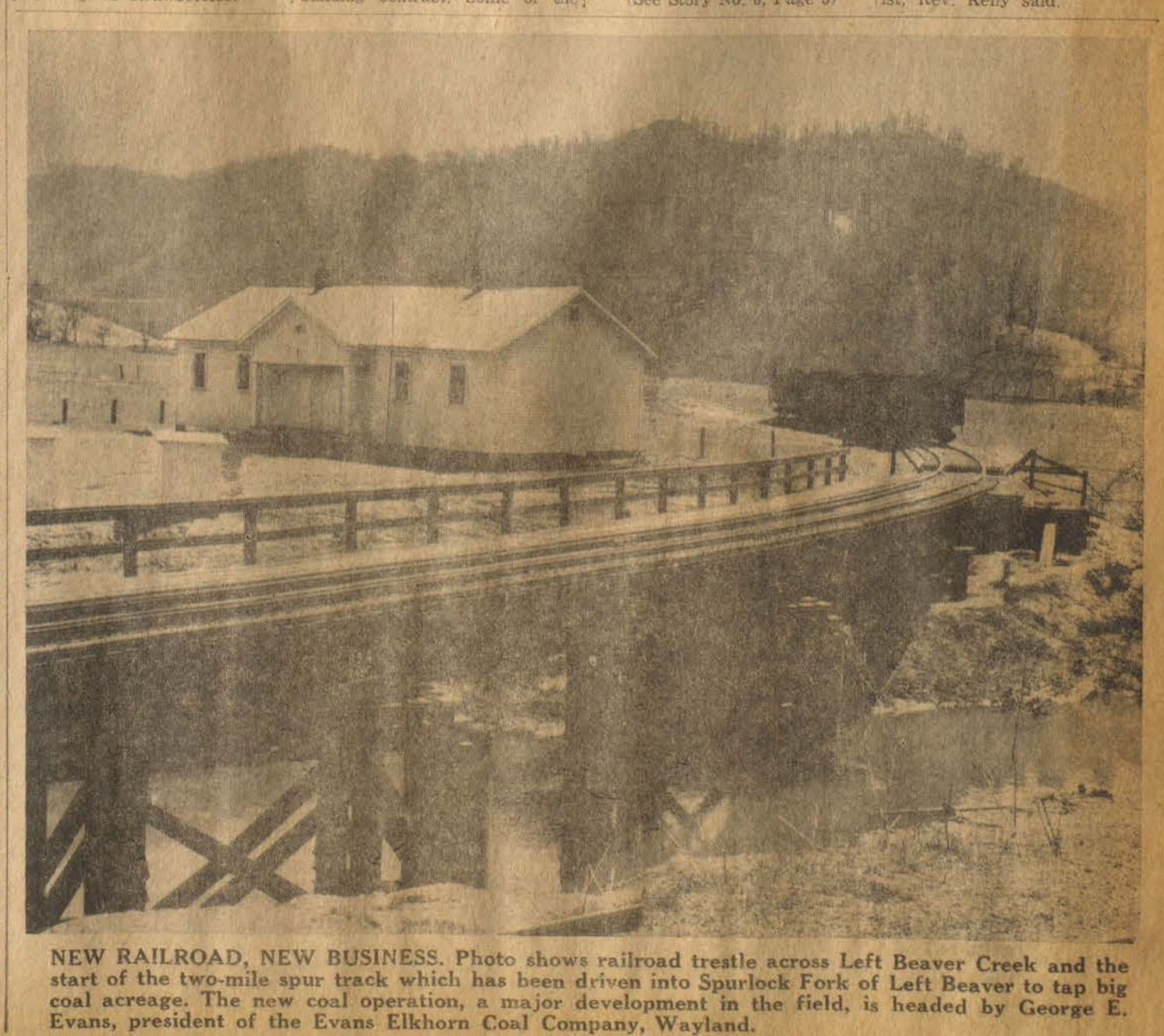
NEW RAILROAD, NEW BUSINESS. Photo shows railroad trestle across Left Beaver Creek and the start of the two-mile spur track which has been driven into Spurlock Fork of Left Beaver to tap big coal acreage. The new coal operation, a major development in the field, is headed by George E. Evans, president of the Evans Elkhorn Coal Company, Wayland.
