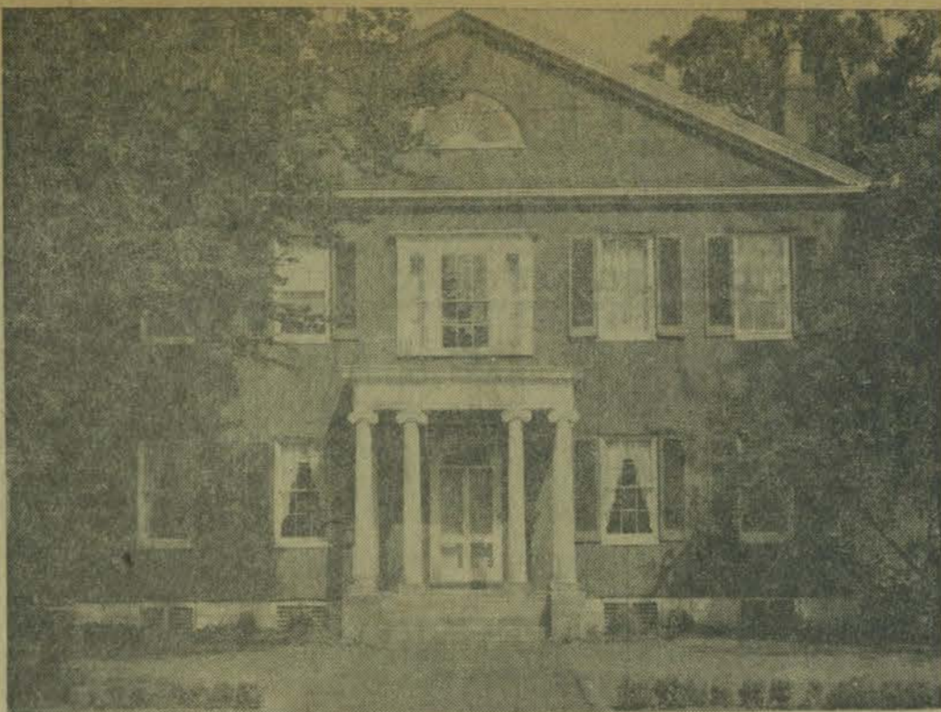
THE ORLANDO BROWN HOUSE in Frankfort was built in 1835 for the staggering sum of $5,000. Designed by Gideon Shryock, an enthusiastic disciple of the Greek Revival style of architecture, the entranceway also reflects the Federal style. At a time when closets were virtually unknown, Brown had a storage room designed off his young wife's bedroom. Brown himself, born in historic Liberty Hall in Frankfort, studied law and medicine and later became editor-publisher of the Frankfort Commonwealth. Until 1955, his descendants occupied the Brown house. Many heirlooms and art treasures still grace the old home, restored and operated by the Colonial Dames of America. Located at Wapping and Wilkinson Streets, it is open from 10 a. m. to 5 p. m. on Tuesday, Wednesday and Saturday and Sunday from 2 to 5 p. m.
