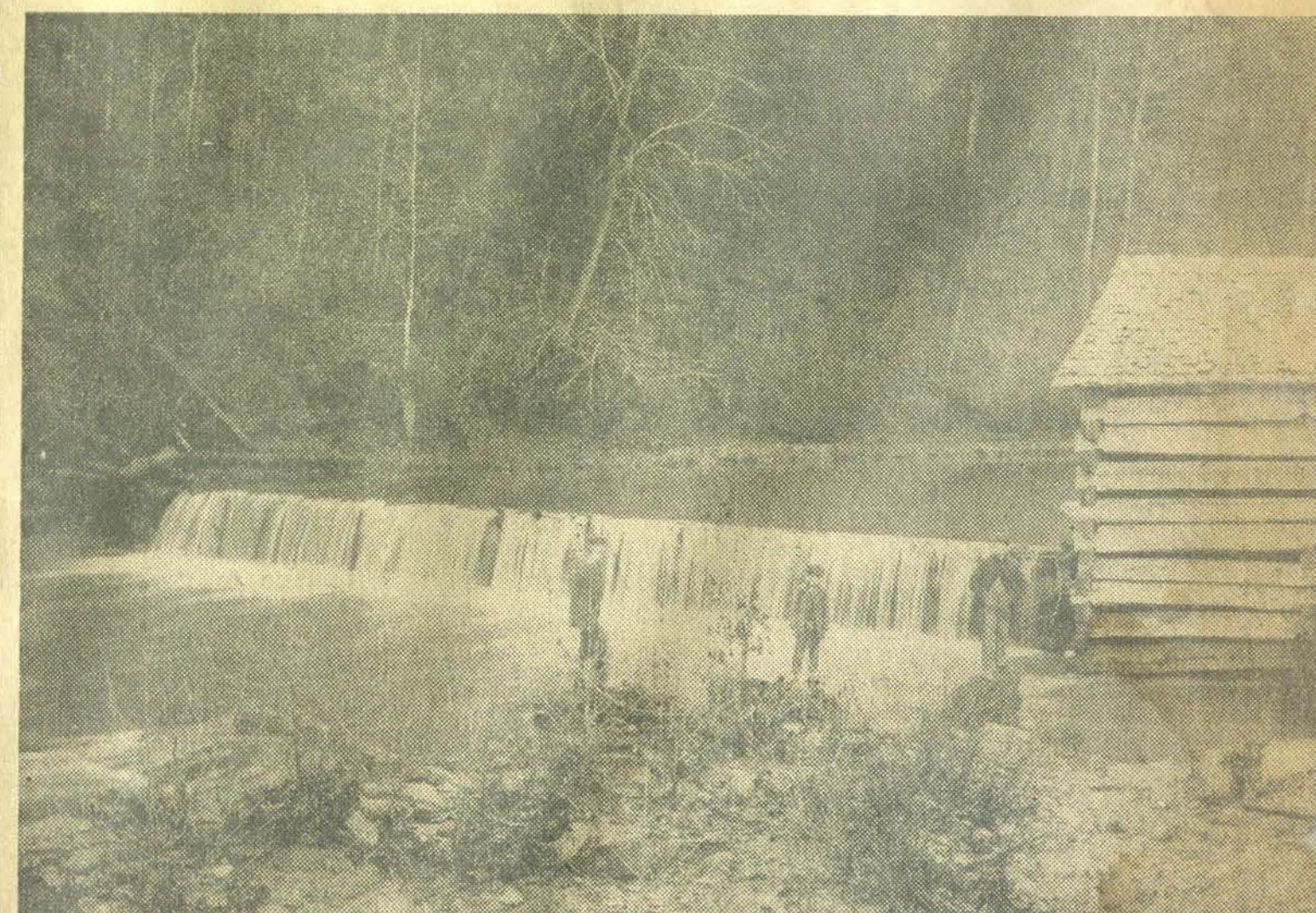
AN OLD MILL DAM OF SIXTY YEARS AGO
