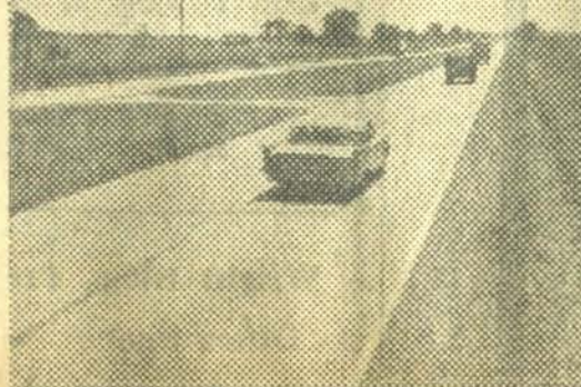
Concrete section on Indiana Test Road, built as part of U.S. 31. After 8 years it is still in fine shape. Asphalt sections have now been resurfaced.
