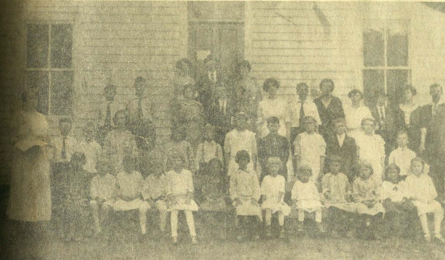
LITTLE PAINT CREEK SCHOOL IN 1916
