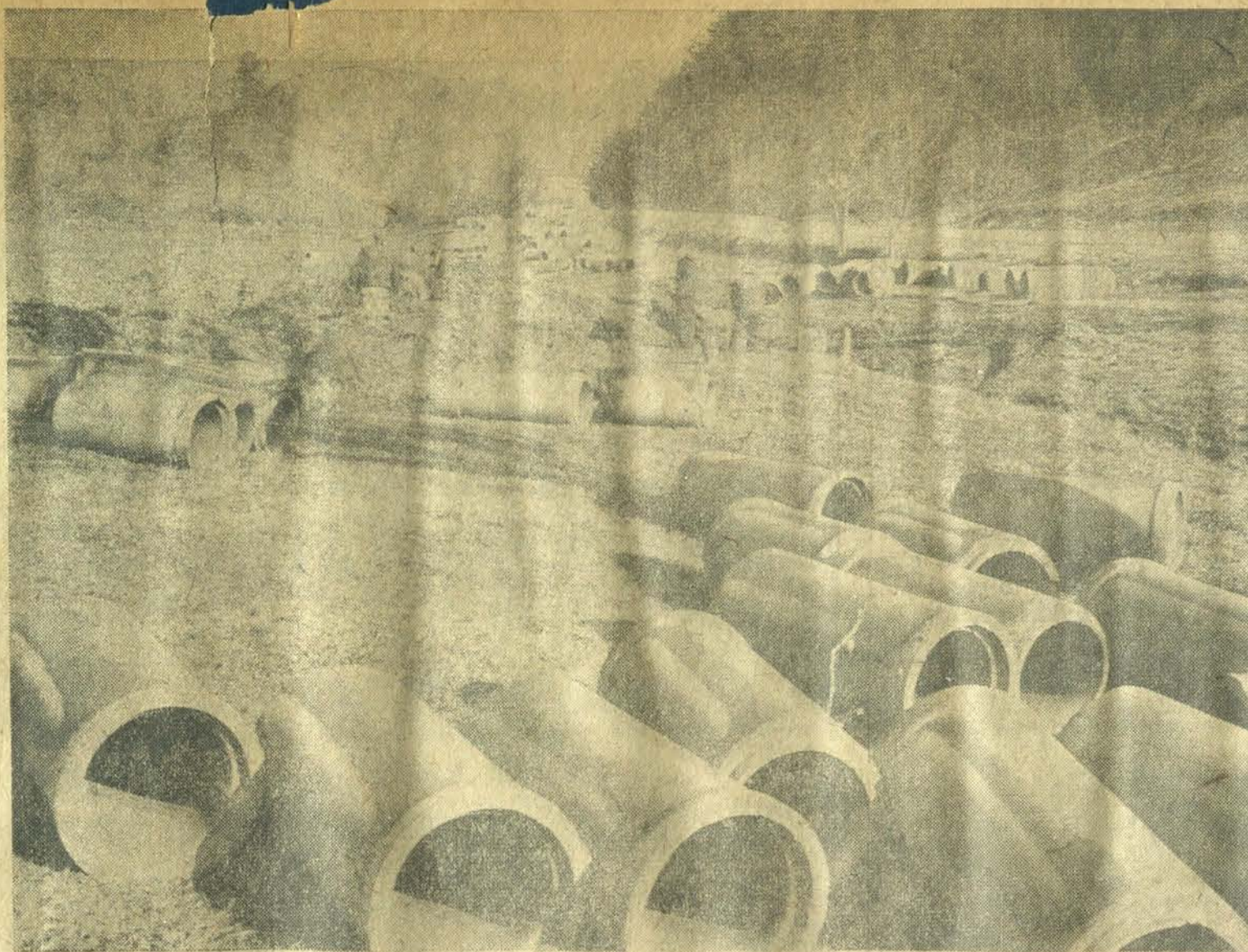
Tile for drainage of the Jenny Wiley State Park's nine-hole golf course is on the ground, waiting drier weather for installation. The golf course work will be under way this spring and summer, but the grass greens are not expected to be playable this year.
