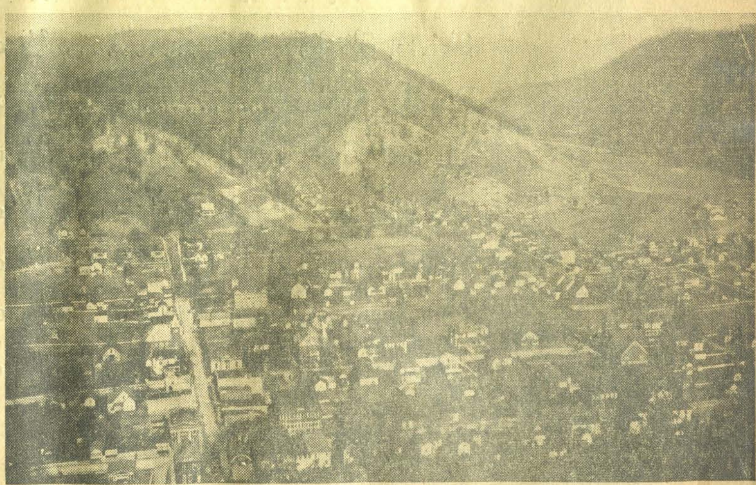
VIEW OF SOUTH PRESTONSBURG FOUR DECADES AGO
