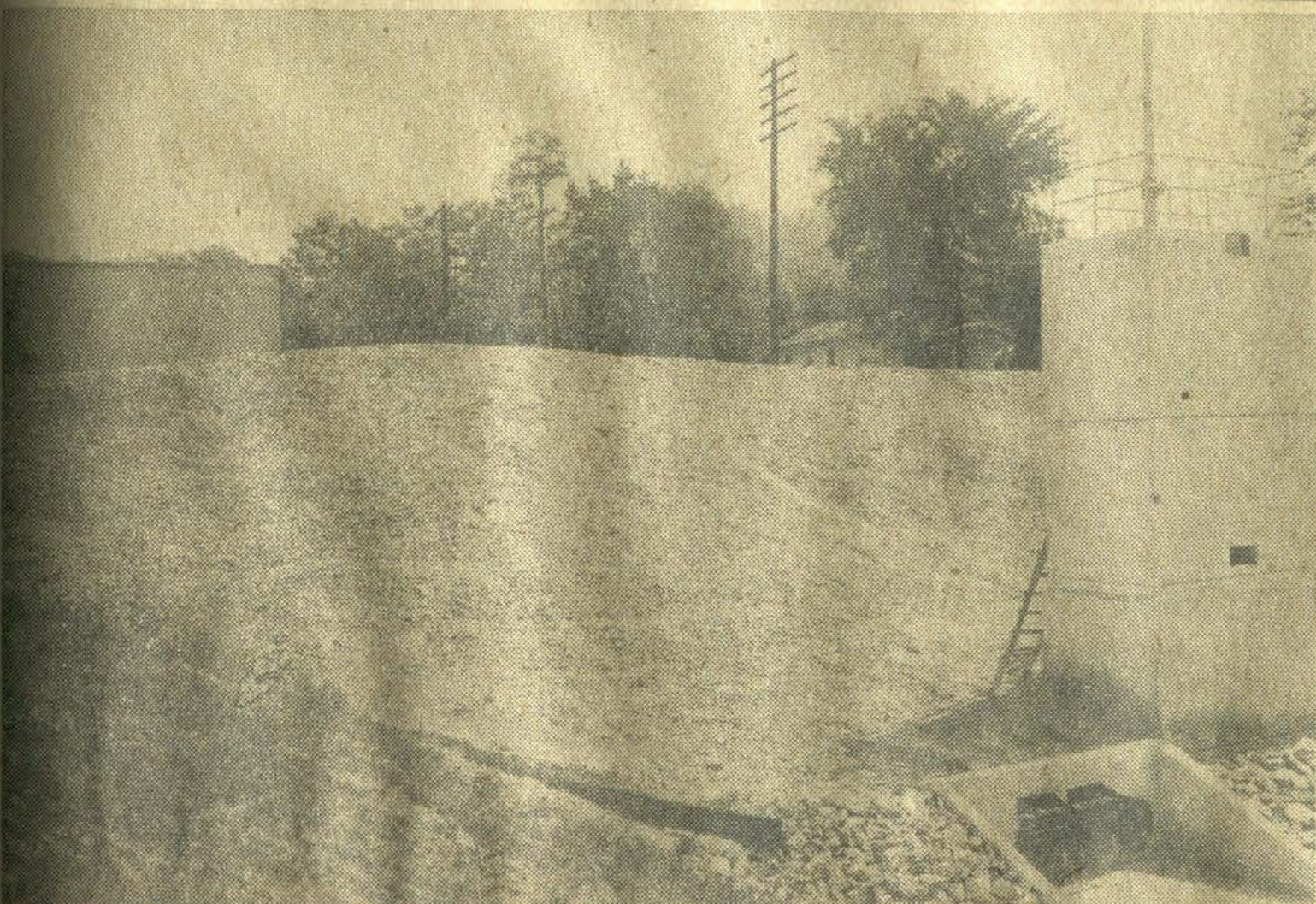
The floodwall that stands between Prestonsburg and the Big Sandy River is now completed. This picture, taken from the riverside, shows the control building and embankment.
