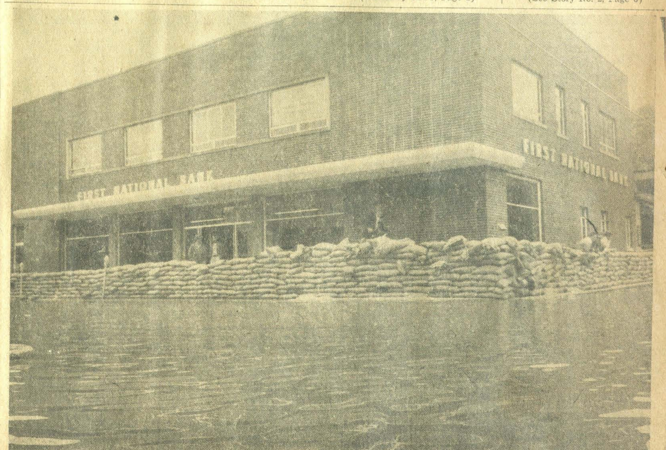
This was the scene last Thursday as the fight to keep the Big Sandy out of the First National Bank here succeeded with the aid of sandbags and pumps. Next day, the bank and other nearby places of business were ready to resume work.
