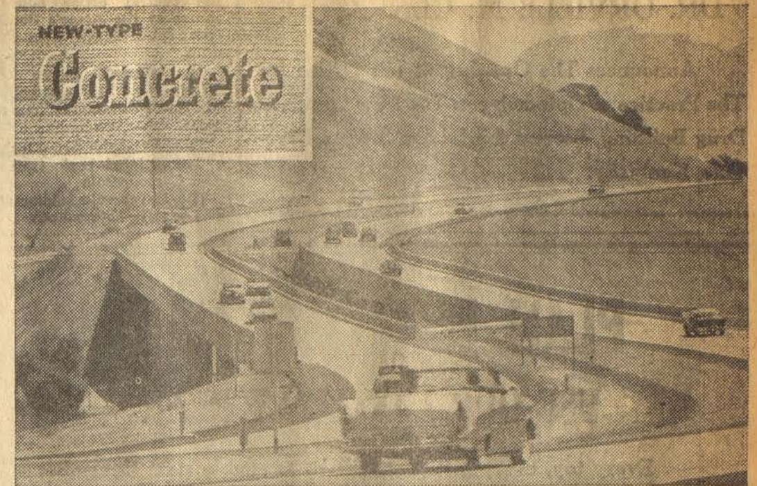
Look of the future on newest highways calls for concrete.
