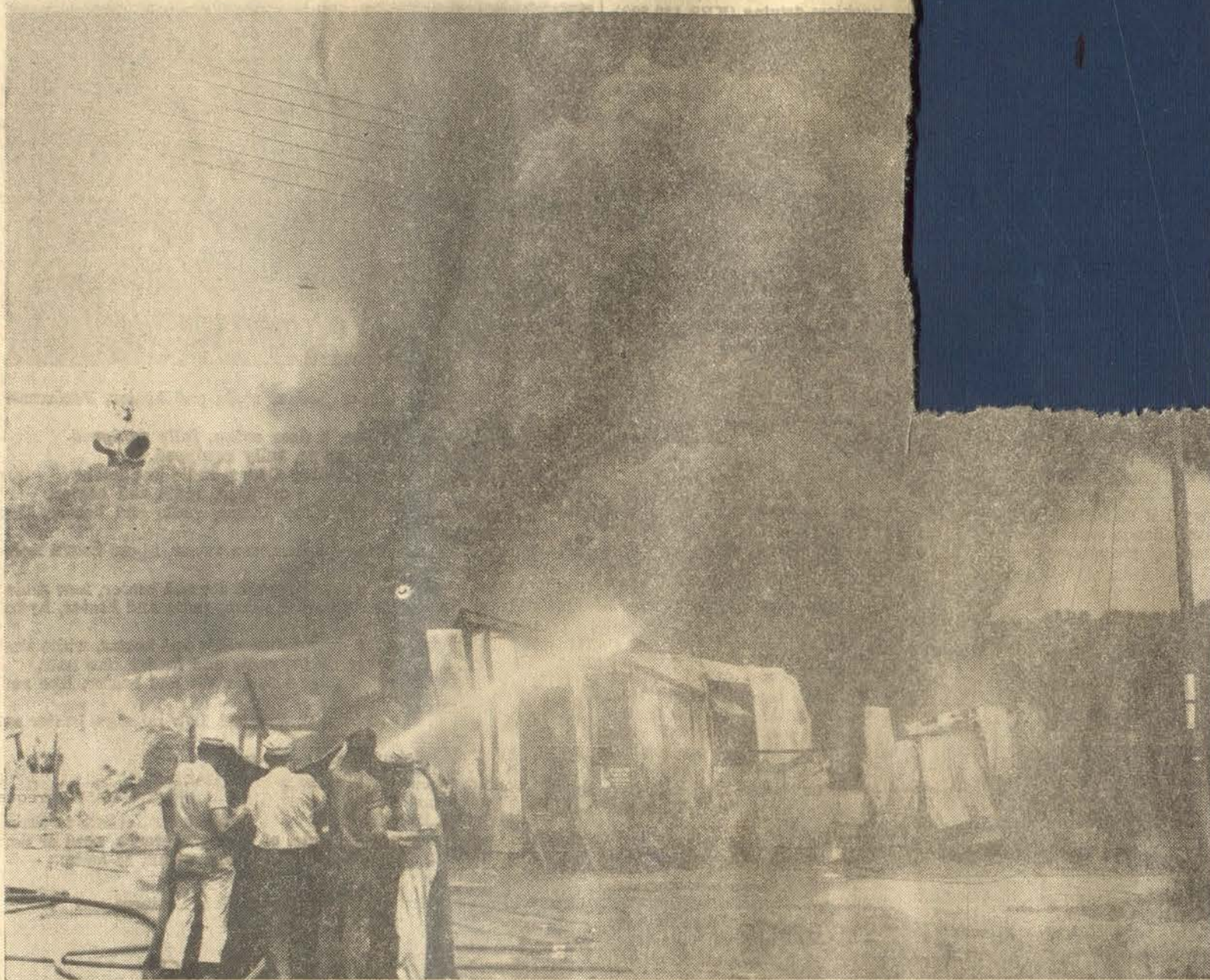
Terrific heat forces firemen to shield themselves as they battle the fire which eventually caused $200,000 damages to Van Hoose Lumber Company in West Prestonsburg. The firemen succeeded in confining the flames to the lumber company and the N. M. White building, except for damages to railroad cars.
