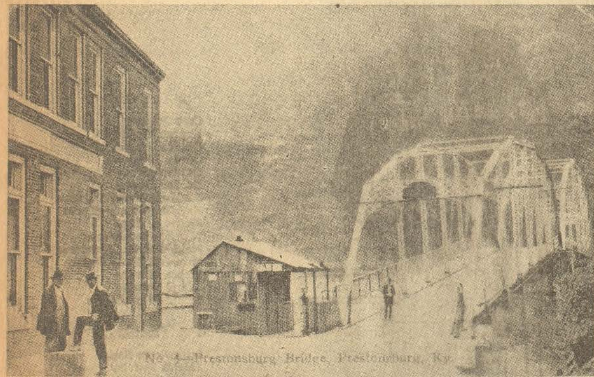
PRESTONSBURG TOLL BRIDGE
