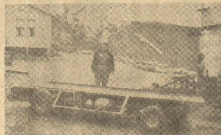
NEW COAL CAR—Pictured is the new coal shuttle car, which is being produced in Pikeville by the Hayes Metal Products of Pikeville. The car, with a capacity of two tons, will sell for about $2,500. A. E. Hayes, June D. Hayes and B. P. Bogardus who own and operate firms at Hi Hat and Richlands, Va., are promoters of the Pikeville firm.
