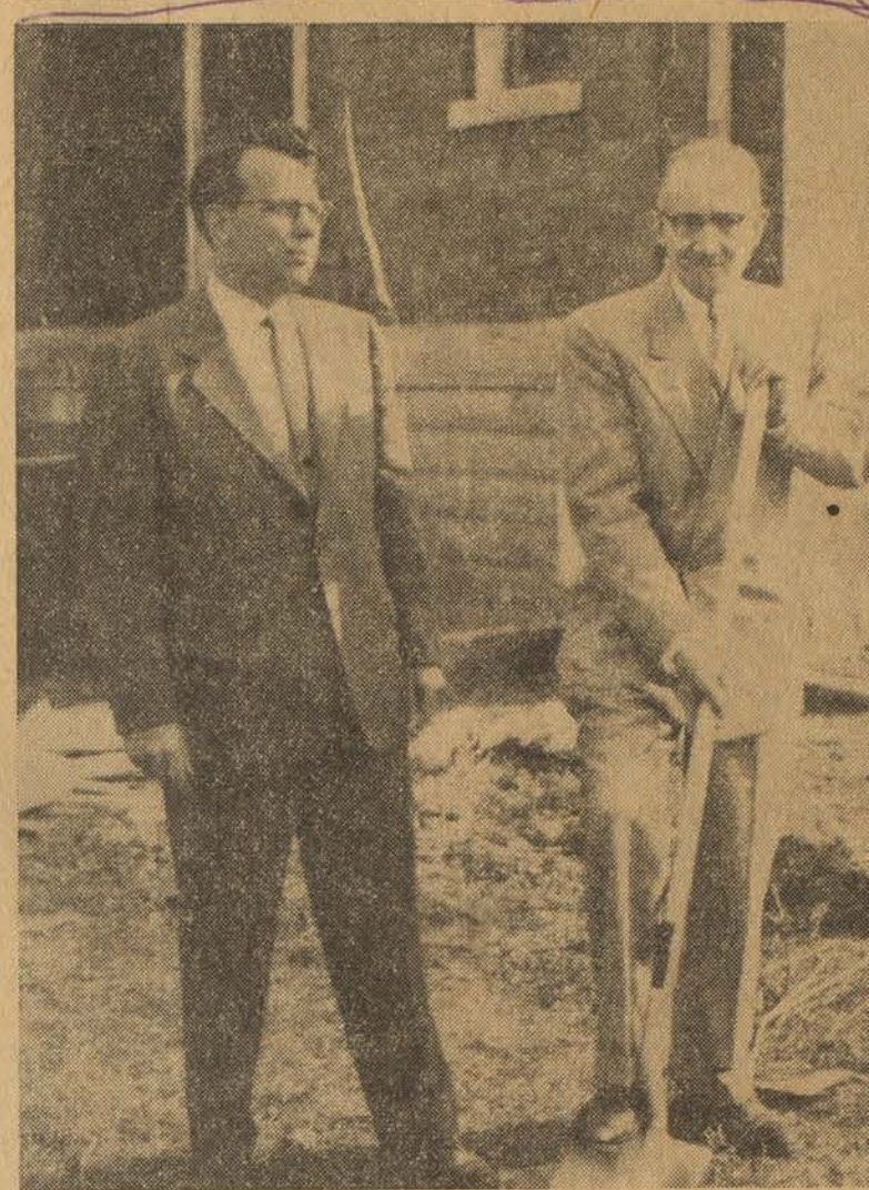
Dr. C. L. Hutsiniller shovels the first earth at ground-breaking ceremonies for the Methodist Church education building here. The Rev. Harold W. Dorsey, pastor of the church, is shown with him.
