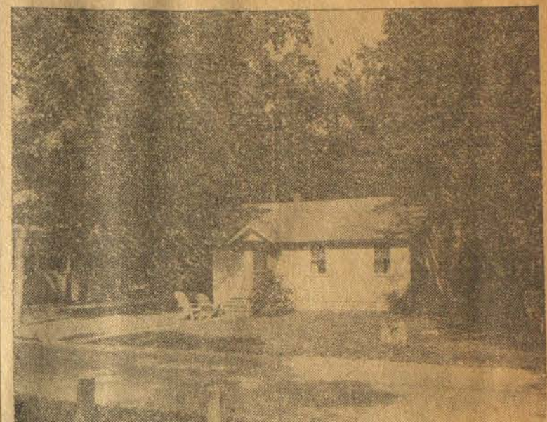
TYPICAL OF THE COTTAGES for vacationists at Kentucky Dam State Park is the one shown above. Each has two bedrooms, a living room, bath and kitchenette. They are available now.
