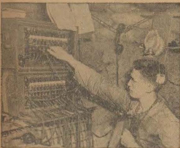
Telephone Switchboard in Dugout in New Guinea — U. S. Army Signal Corps Photo
