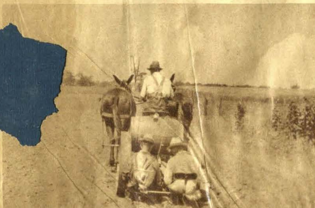
Setting tobacco with machine setter
