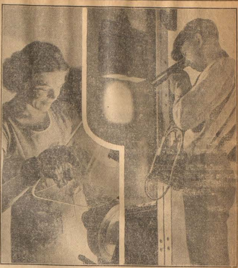
THAT'S what Consumers Information calls these workers in a Pittsburgh glass plant, who are testing and finishing non-shatterable glass for use in automobiles. It is explained that one of the greatest hazards in auto accidents used to be flying glass, which was the most common cause of injury. Now all American cars are equipped with the shatter-proof variety, developed by American industrial research experts especially for this purpose, and the saving of many lives is the result. The man shown above keeps a constant vigil with his pyrometer, to assure proper melting conditions. The girl is polishing the edges of a car window.
