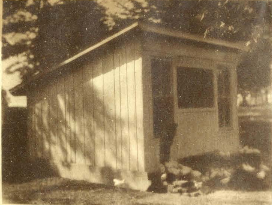
A CHICKEN HOUSE ON SKIDS—Here is a brooder house that can be moved on new skids to afford new grounds for growing chicks. The picture was made on the poultry grounds of the University of Tennessee Farm.
