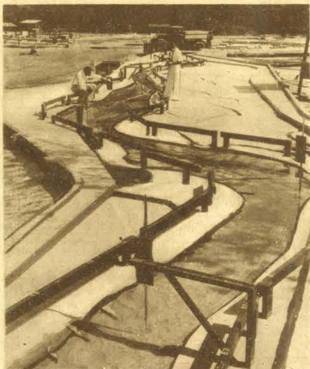
OLD MAN RIVER in miniature, rampages and all, is constructed by the U. S. Army Engineers at Vicksburg, Va., to learn vital flood control lessons. The laboratory covers 225 acres and includes an 80-acre lake. (Acme)
