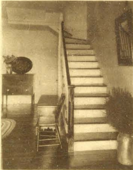
An enclosed stairway opened, a rail substituted for a partition, and floor refinished modernize the old Peter Gann home.
