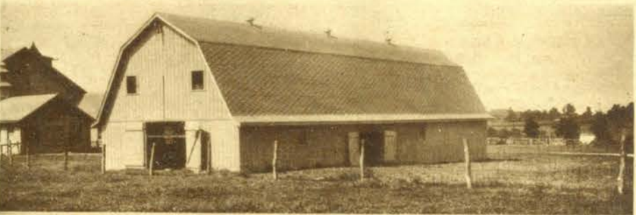
Hip-roof replaces gable on this barn.
