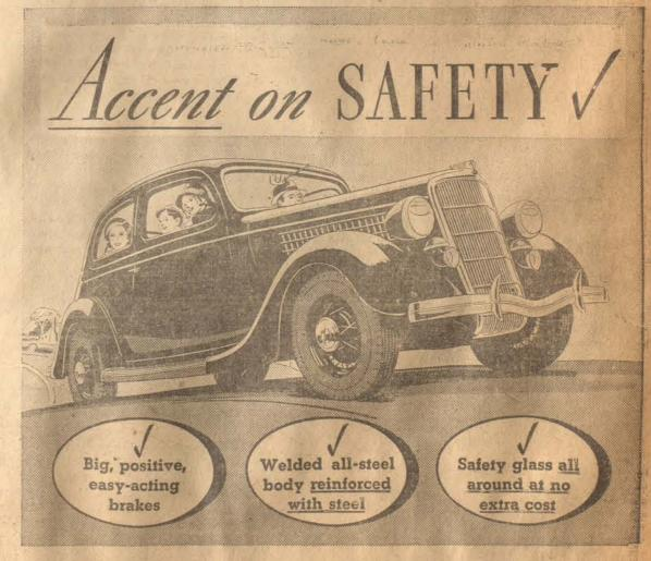
THE 1935 V-8 is the safest Ford car ever built. A Safety glass is standard all around in every model, at no extra cost. Ford bodies are all-steel, welded. The Ford double channel X-type frame is low, rigid, strong.
