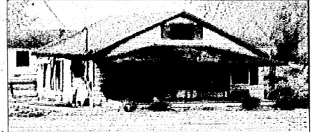
This Lancer home burned Friday night, despite being vacant and having no electricity. The fifth fire in the immediate area over the past few months, officials are now considering the possibility of arson.
