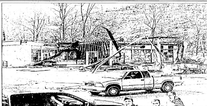
The Marathon station at the beginning of the Mountain Parkway was completely destroyed.
