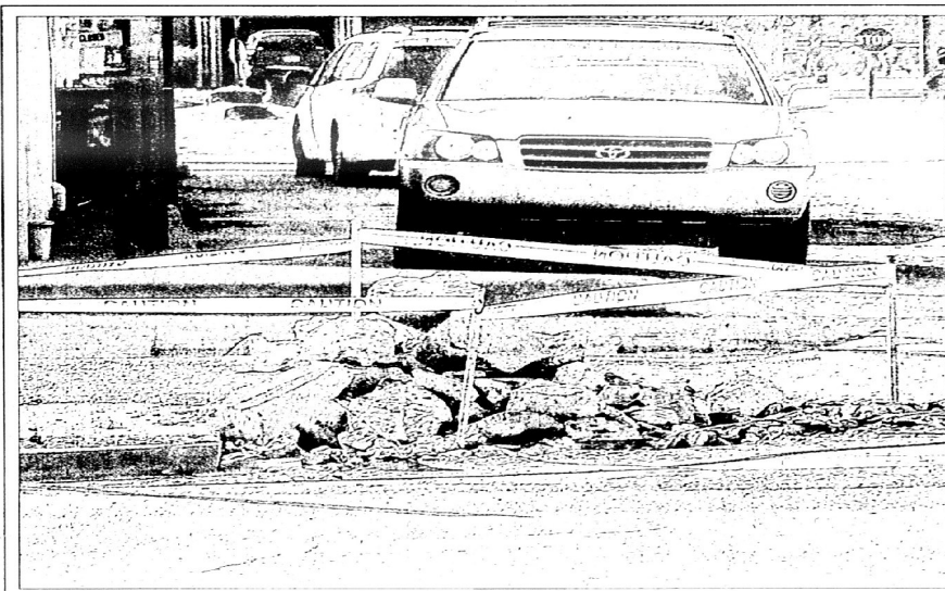
There has been some noticeable construction in the city of Prestonsburg lately, as crews work to improve sidewalks to make them more handicapped and stroller friendly. photo by Jack Latta
