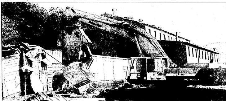
Demolition work began at the Kentucky West Virginia Gas complex in Prestonsburg on Wednesday. According to Fire Chief Bobby Carpenter, there are several options for the land, from restaurants to office buildings. The main Kentucky West Virginia Gas building is scheduled for demolition as soon as asbestos workers complete their inspection. Carpenter said the demolition on the main building could begin in 1-to-2 weeks.
