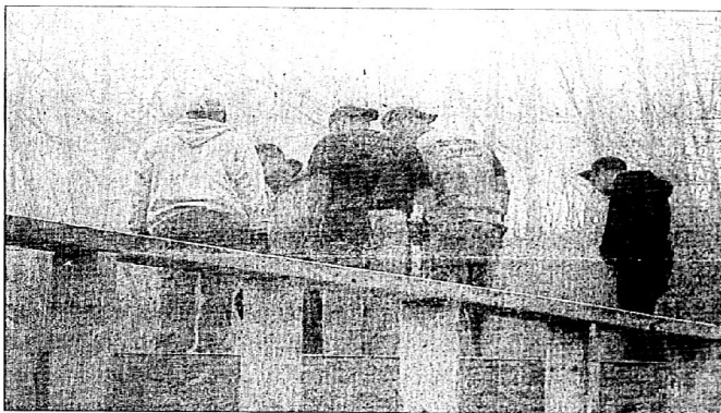
Big Sandy Community and Technical College students Justin Robinson and Roger Bowling joined volunteers from the WestCare Foundation in helping construct a Habitat for Humanity home in Pikeville.
