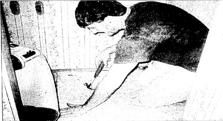
Workers with the Big Sandy Area Community Action Program weatherization crew recently completed work on a Printer home, replacing skirting and floors and installing a new heat pump, floor insulation, smoke and carbon monoxide detectors, window caulking and two new doors.
