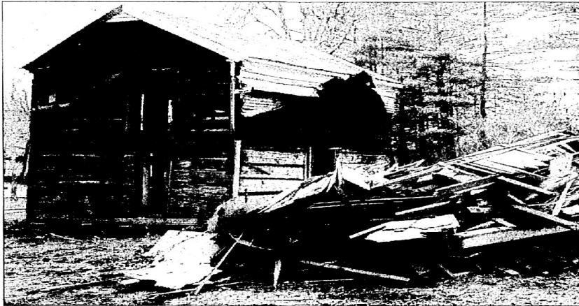
This two-story cabin just off Mays Branch Road, which dates back to the mid-1800s, according to owner Bobby Ray White, will soon be sold to the highest bidder. White recently tore down the additions that had been built around the historic home to reveal the original structure. The home might have once functioned as a birthing house where midwives helped women through labor and could, according to some local historians, pre-date the nearby Samuel May House. The last section added had been built around the structure in the 1950s by White's father.
