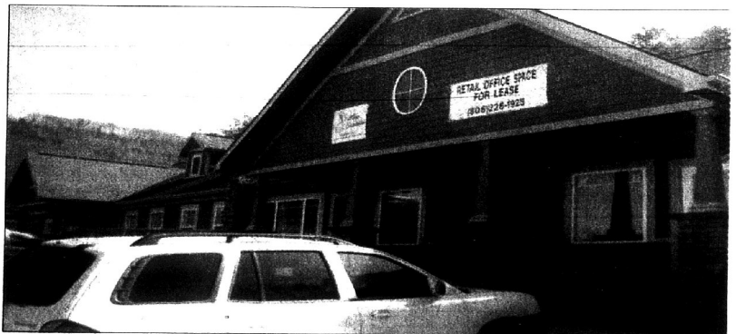
Village Boutique has been in its current Prestonsburg location near the entrance to Stonecrest for three weeks.
