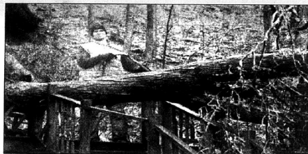
Michael Brown starts the long task of clearing away a large tree that fell across the porch of his family's home along Lakeview Village Road Wednesday. Lakeview was one of the hardest hit areas of Floyd County following the worst ice and snow storm in more than a decade.
