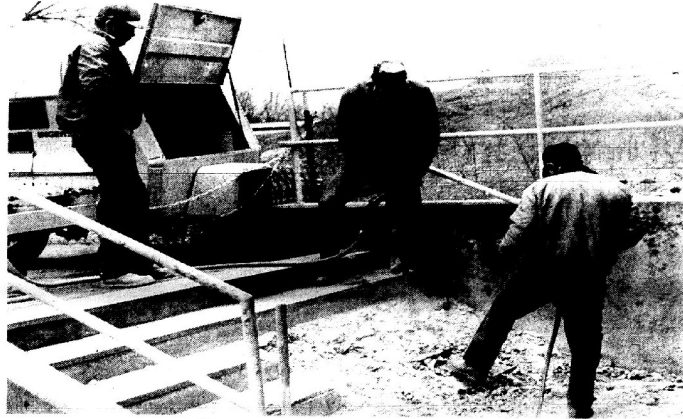
Ramp construction underway Floyd County school maintenance workers began constructing a wheelchair ramp Thursday at the Betsy Layne gym. Betty Keathley of Allen has been trying to get a ramp built at the gym for the last two years. Her son, Danny, was injured in a coal mining accident and is confined to a wheelchair. Danny Keathley goes to the gym to watch his son play basketball. (photo by Terry Spears)
