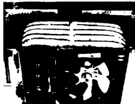
With units that have fins, despite their comb-like appearance, do not attempt to straighten them.
