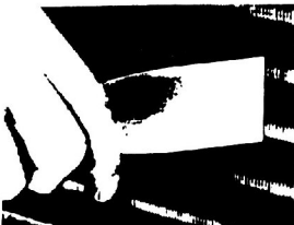
Use a putty knife to restore the space between fins. No two fins should touch one another.
