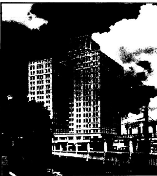
The Milam Building, opened in 1928 in San Antonio, Texas, was the nation's first high-rise, air-conditioned office building. The Milam Grill hosted daily luncheon crowds seeking its cool comfort.
